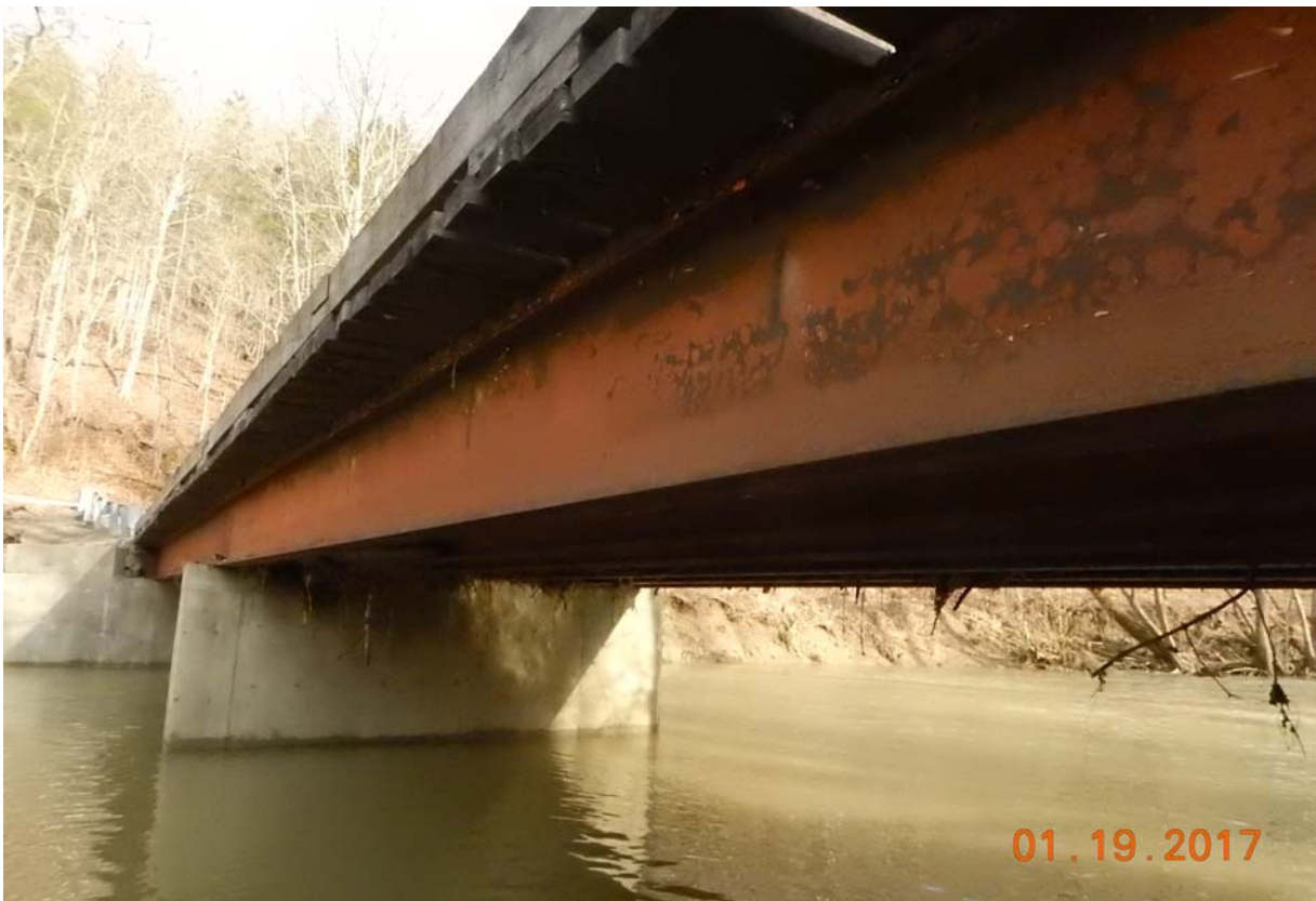
View of the east span.
