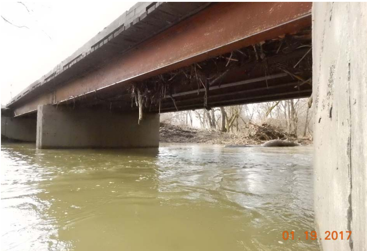
View of the underside of the west span.
