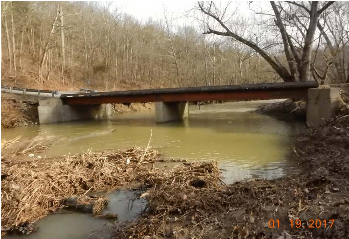
View looking at bridge from downstream.
