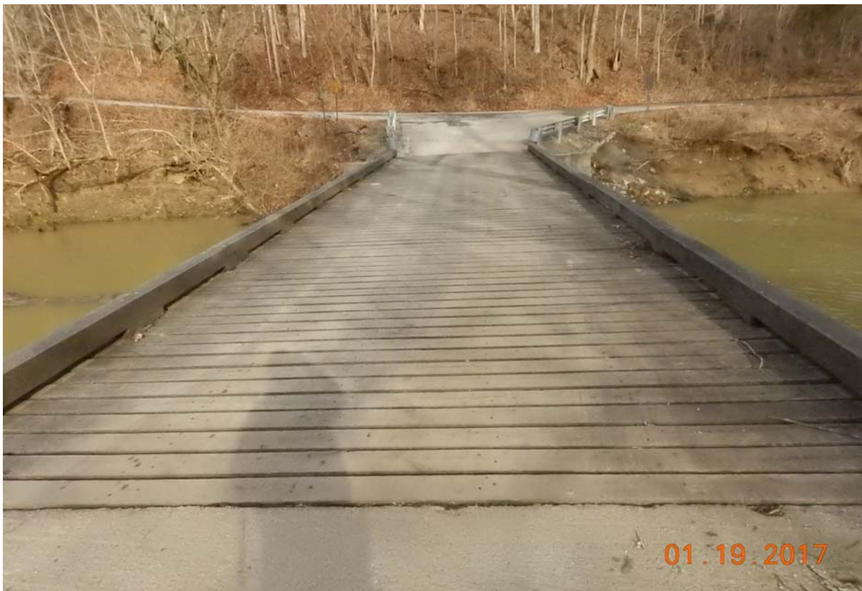
View of the timber wearing surface.
