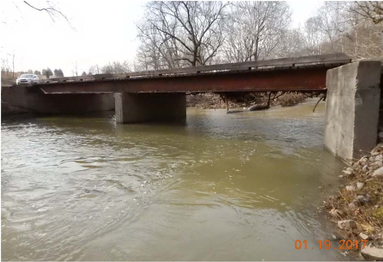
View of bridge from upstream.
